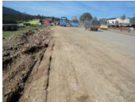
Ongoing road rehabilitation
