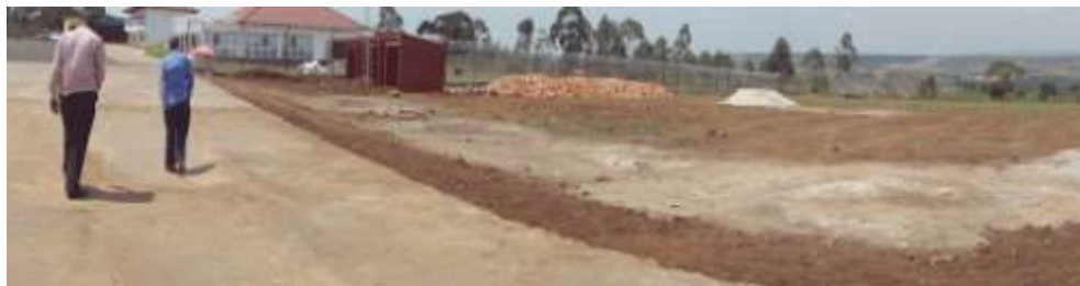
Fig: General view of the RSS from the Main road.
