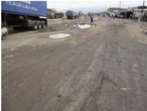
Fig: The parking becomes wet and unusable in wet weather making lorries to park by the roadside.
