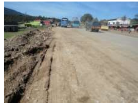
Site clearance for the side parking
