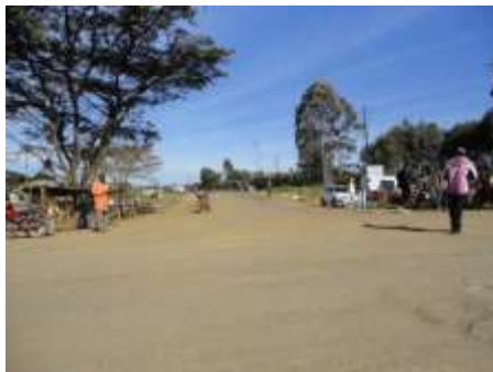
The rehabilitated road to Muhoroni
