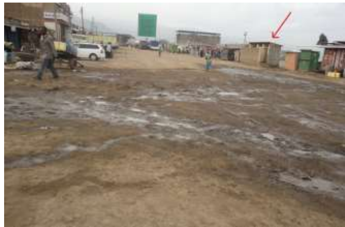
(c) Drainage challenges, with the existing public toilet near the park marked with an arrow
