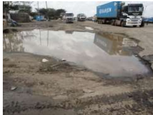
Fig: The parking becomes wet and unusable in wet weather making lorries to park by the roadside.
