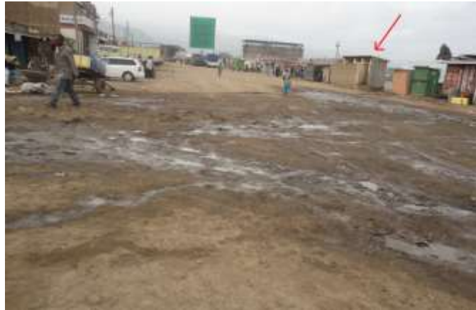
Fig: Drainage challenges, with the existing public toilet near the park marked with an arrow
