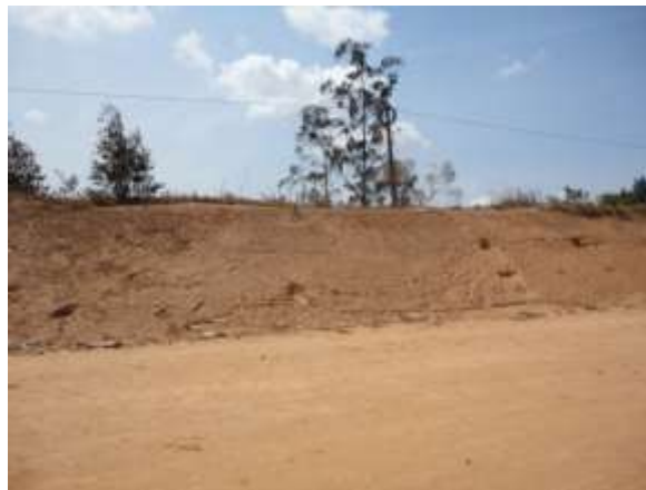
Fig: The western edge of the road where cutting was done
